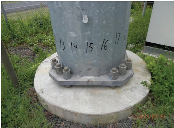
Figure 5. Toe cracks in polygonal poles typically first occur near the vertices (bend-lines or points of the multisided shaft) because this area generally has a higher stress concentration.
