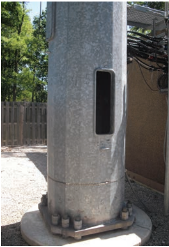
Typical communications monopole base connection
