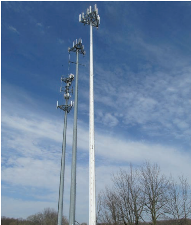
Figure 1. Tubular steel monopoles are popular support structures in many industries. They have seen use as support structures in the communications, sports lighting, utility and transportation industries for many decades.
